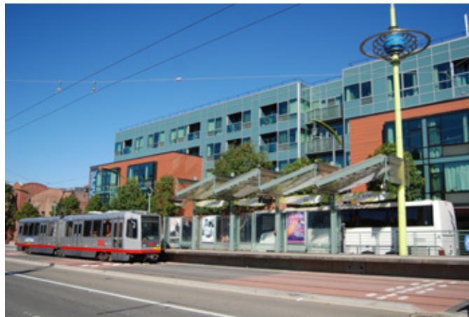
Potrero Launch, San Francisco. Twenty percent of the 196 loft units are affordable to households making between 30 and 50 percent of the Area Median Income. The higher affordability levels were in part the result of the zoning change from industrial to mixed-use which, under the EN plan, called for higher inclusionary housing requirements. Photo courtesy Nico Calavita.
