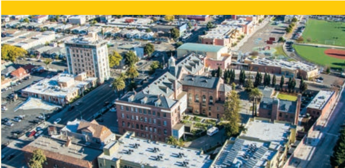
St. Joseph’s, an affordable housing property on a transit-rich corridor in Oakland, is the type of development that can preserve opportunity for residents.
